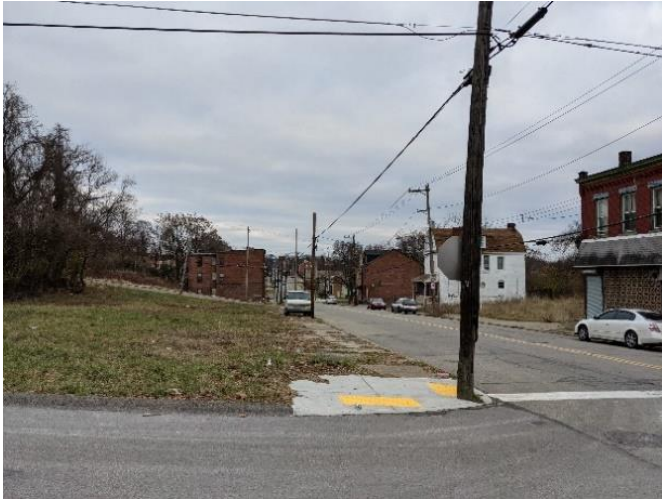
Figure 18. Missing Sidewalk Connection to Curb Ramp
