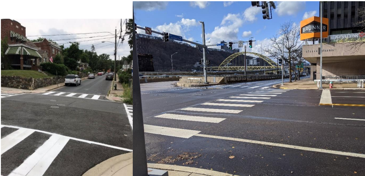
Figure 45 High Visibility Crosswalk traversing Stanwix Street at Fort Pitt Boulevard, Pittsburgh.
