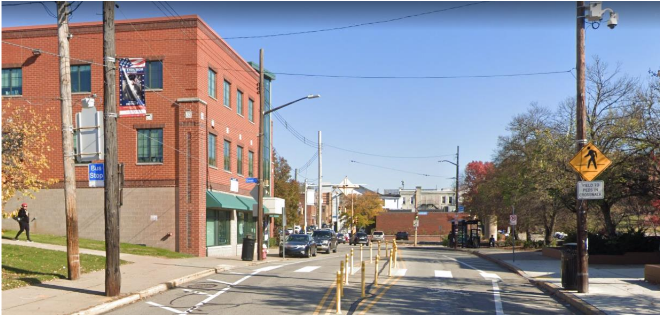
Figure 5. Centre Avenue at Green Street Pedestrian Walkway
