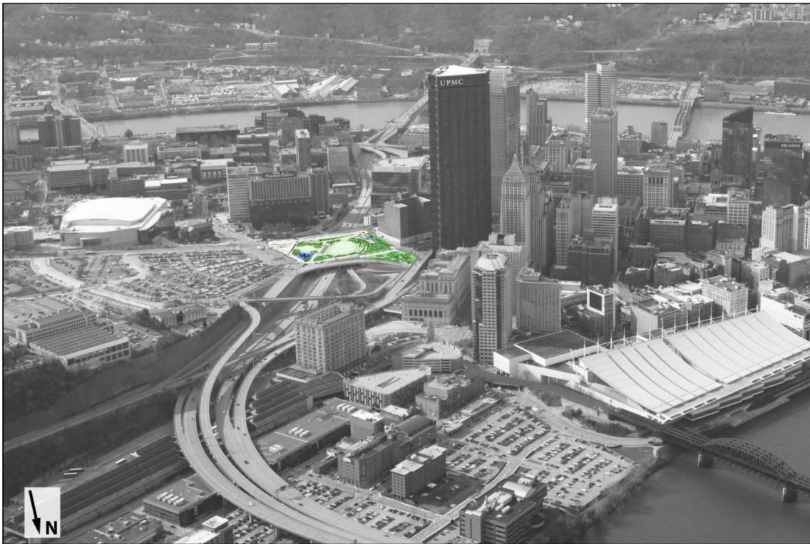
Figure 3. The I-579 "Cap" Urban Connector Project, currently under construction, will help re-connect the Hill District to Downtown
