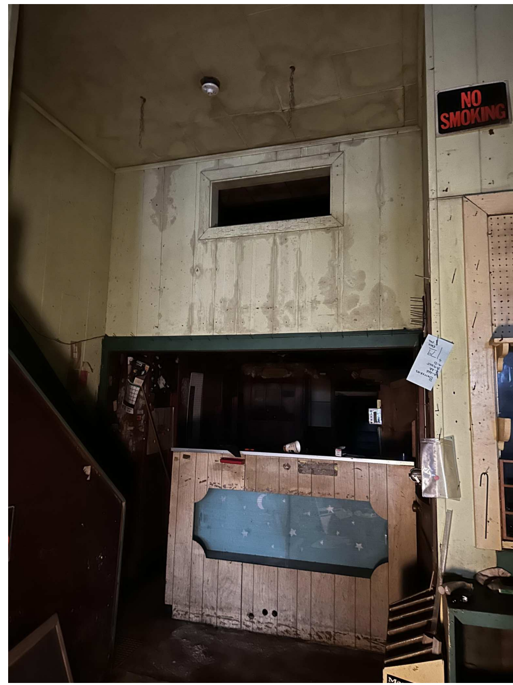
LEVEL 1 DEMOLISH INTERIOR NON STRUCTURAL WALLS, FINISHES, LIGHTS AND BULK HEADS.
