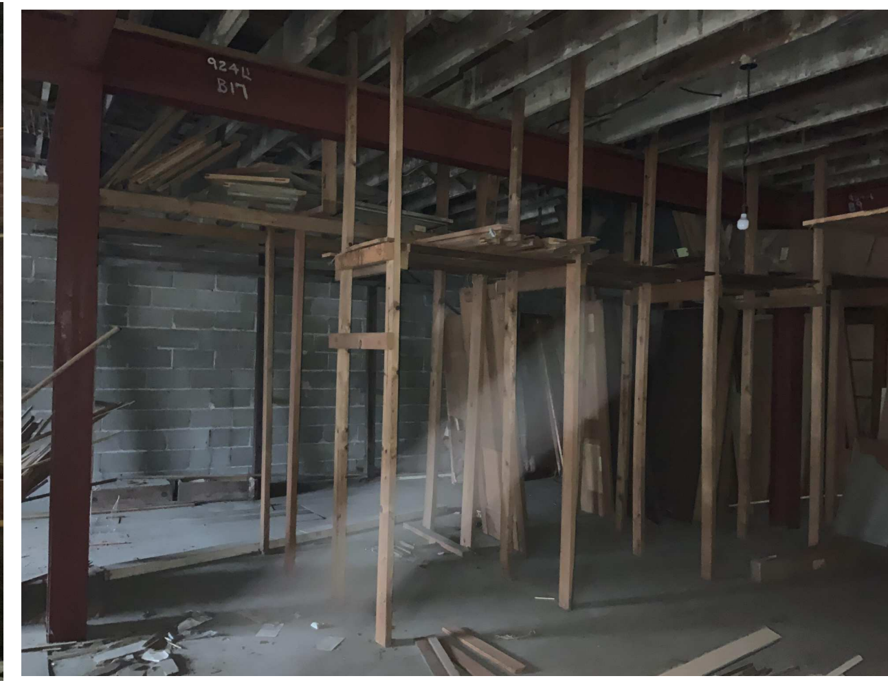
LEVEL 3 DEMOLISH INTERIOR FINISHES AND WOOD FRAMES
