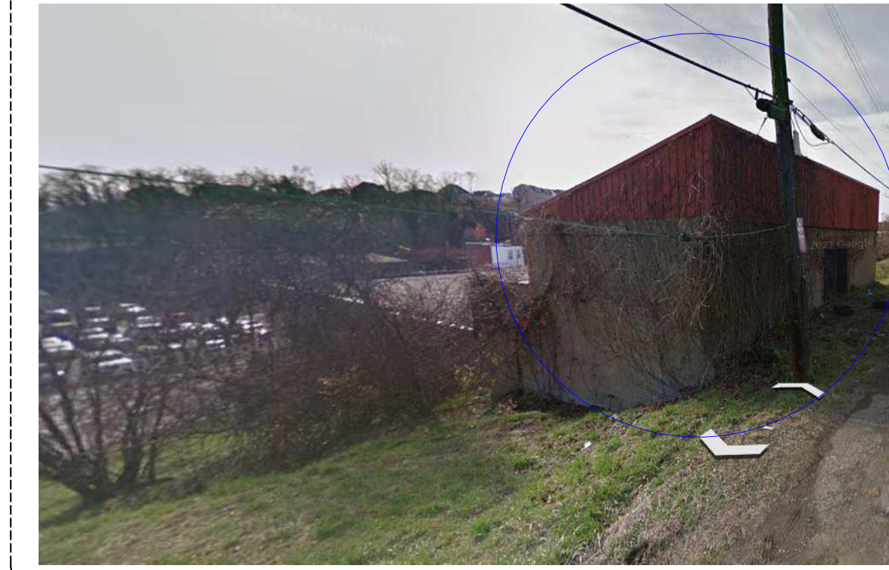
LEVEL 3 DEMOLISH STRUCTURE
