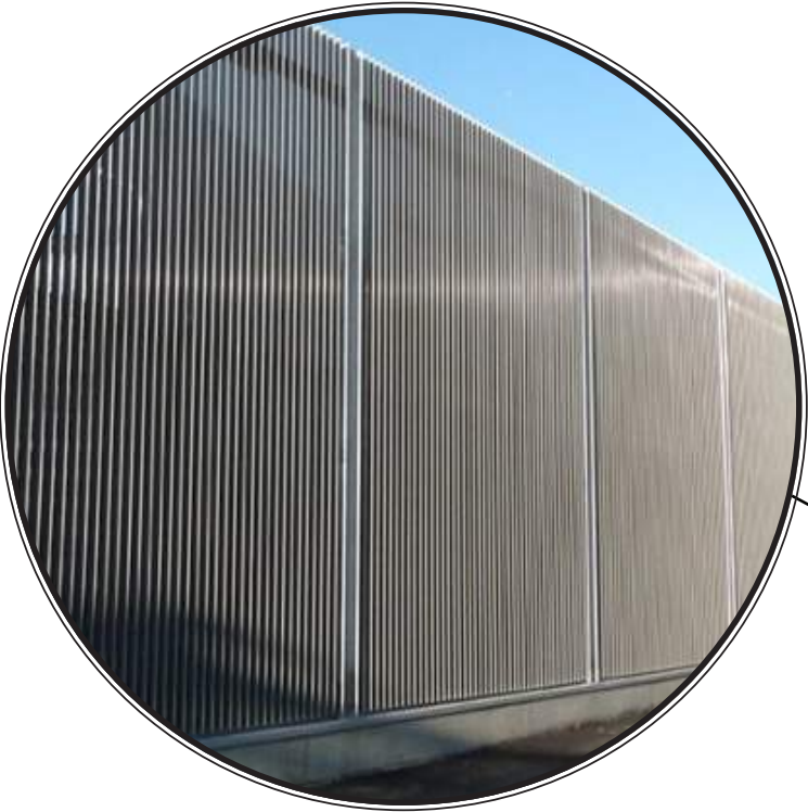
louvered facade for ventilation at parking levels 03+04
