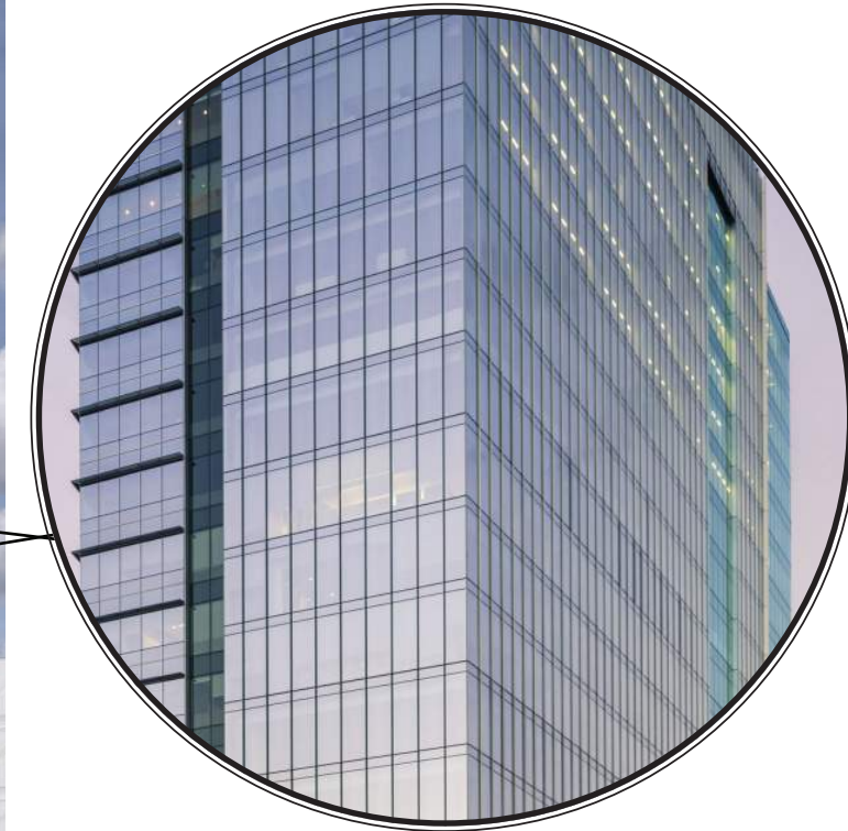
curtainwall with mullion "fin" extensions
