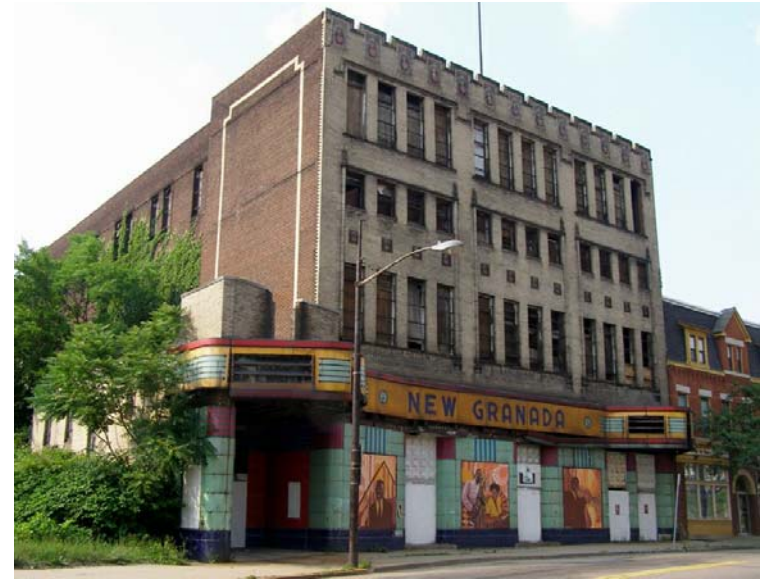
④ CENTRE AVENUE (2000's)
