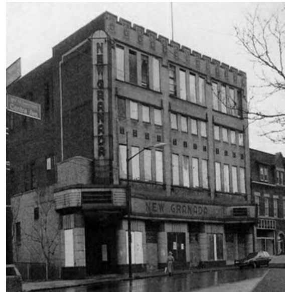
③ CENTRE AVENUE (1990's)
