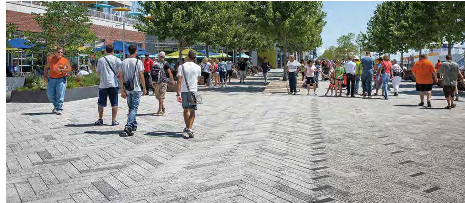
Plank Unit Paving (Mix of Greys/Finishes)
