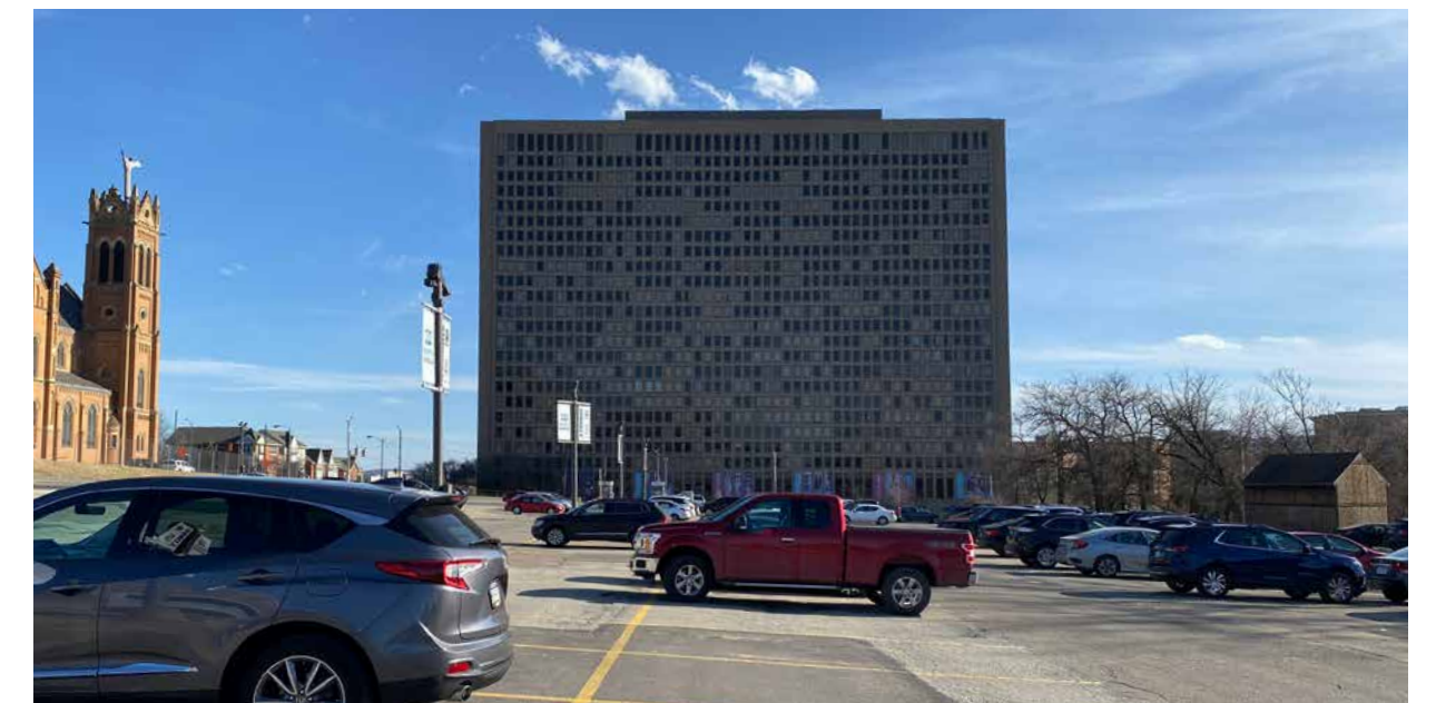
IMAGE 5 View from corner of Wylie Ave & Crawford St
