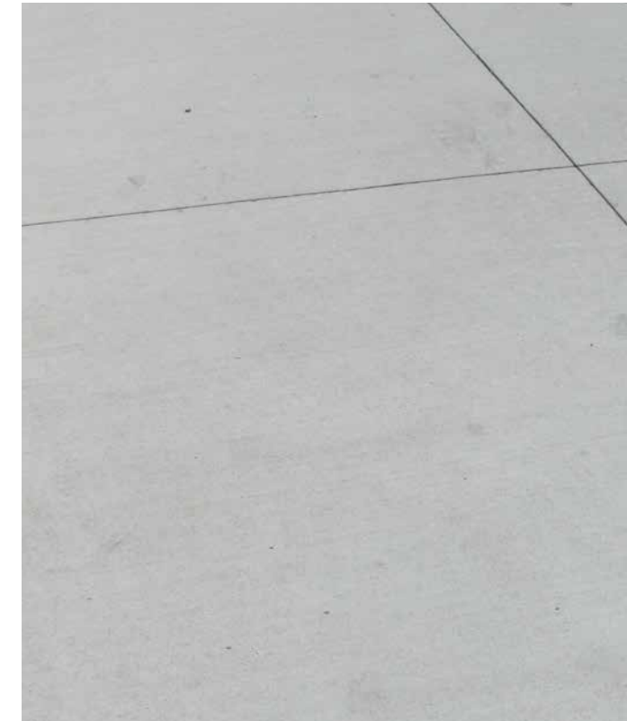
Broom Finish Concrete
