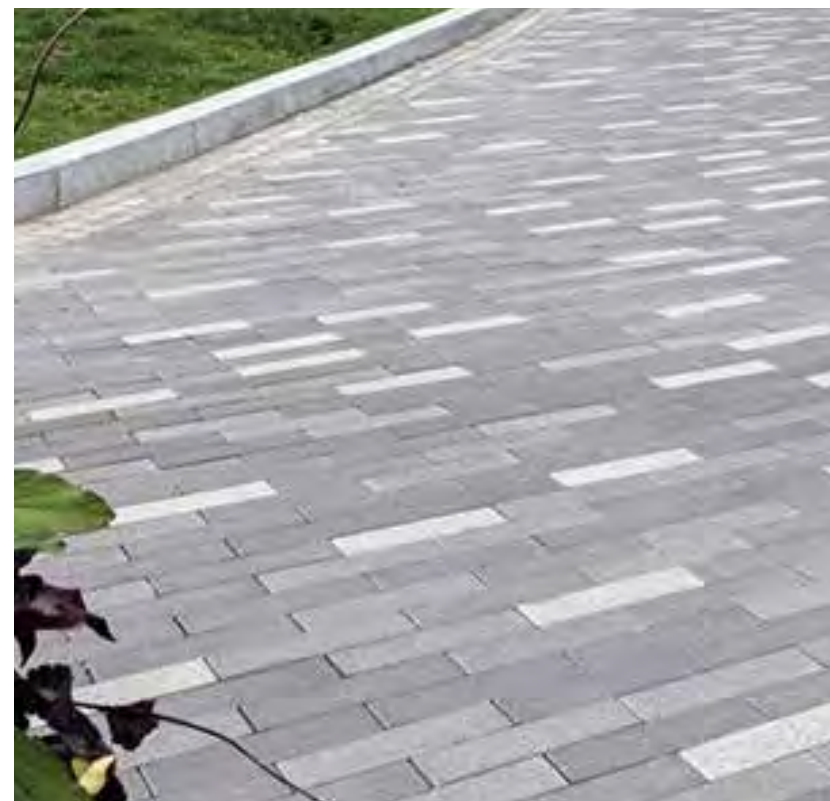
Plank Unit Paving
