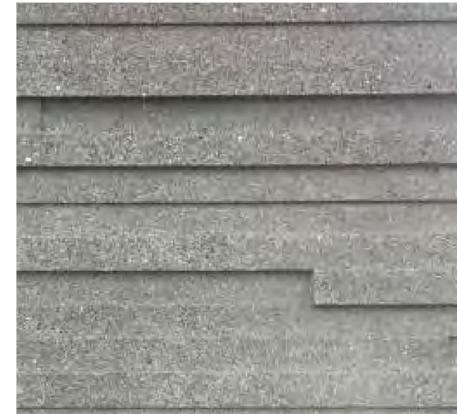
Concrete Wall - Board Form Finish
