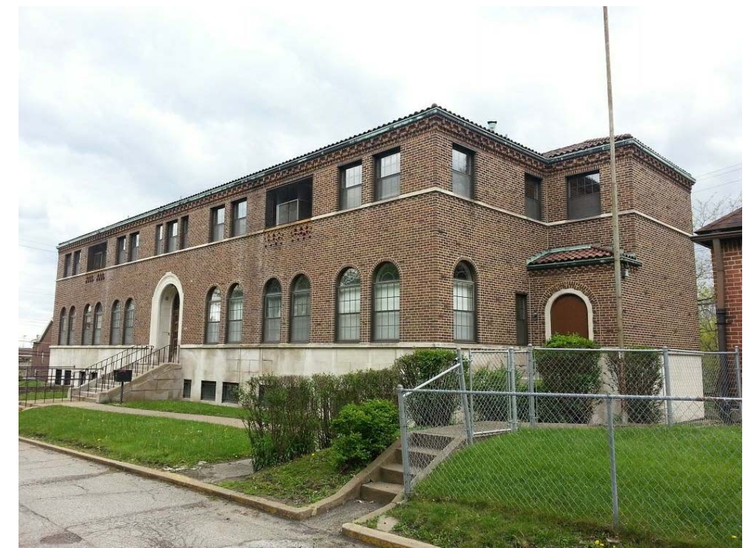
③ FRONT VIEWED FROM NORTH - EAST
