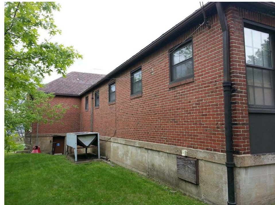
3 REAR VIEWED FROM SOUTH - WEST
