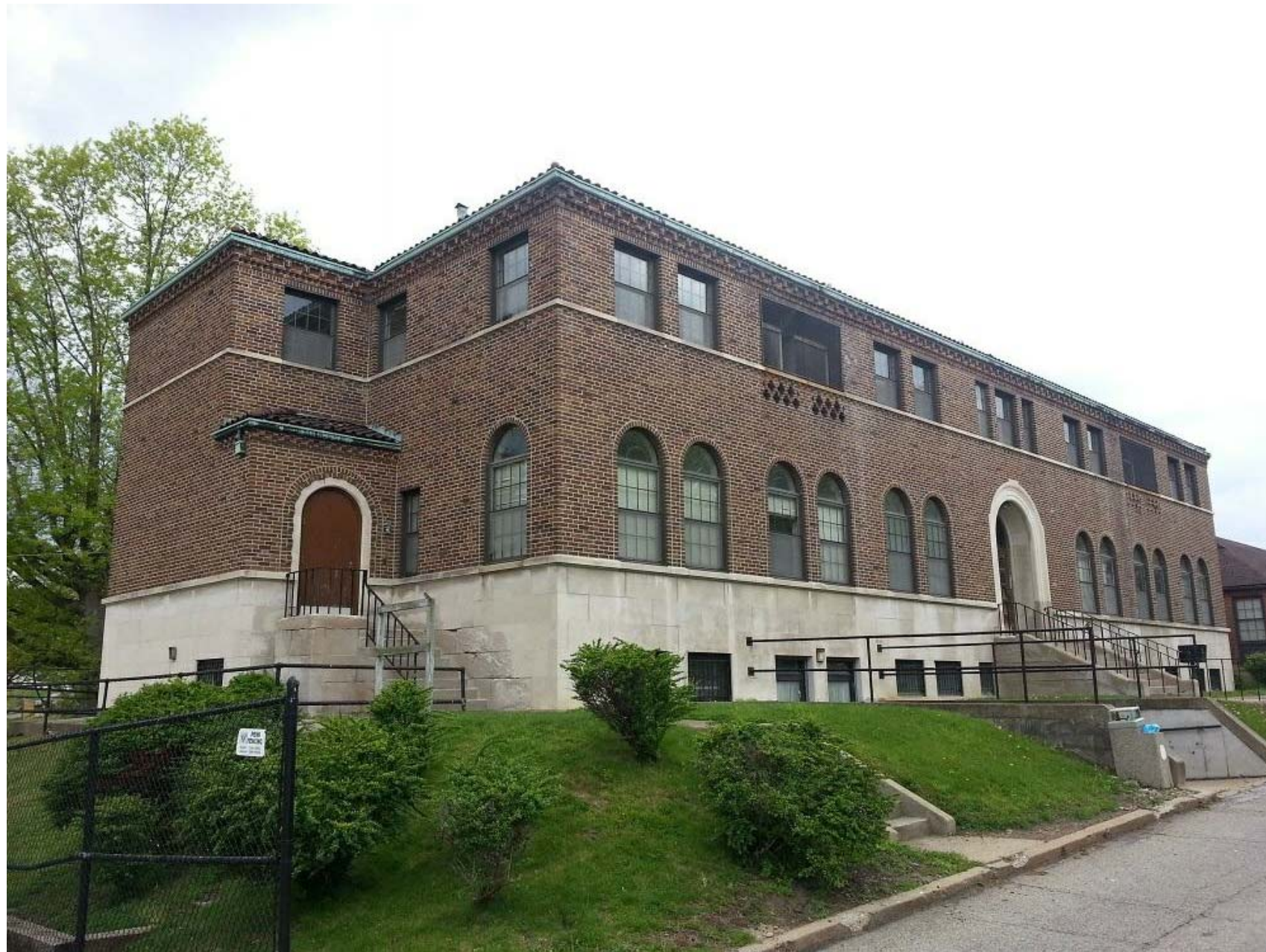
① FRONT VIEWED FROM BEDFORD AVENUE
