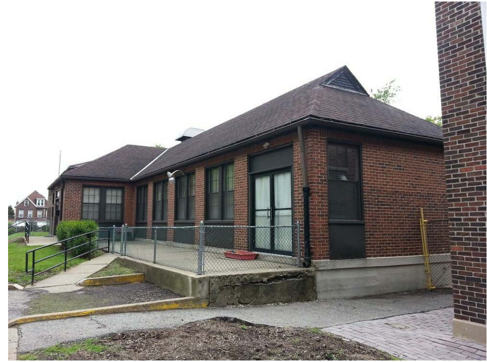
2 FRONT VIEWED FROM NORTH - EAST
