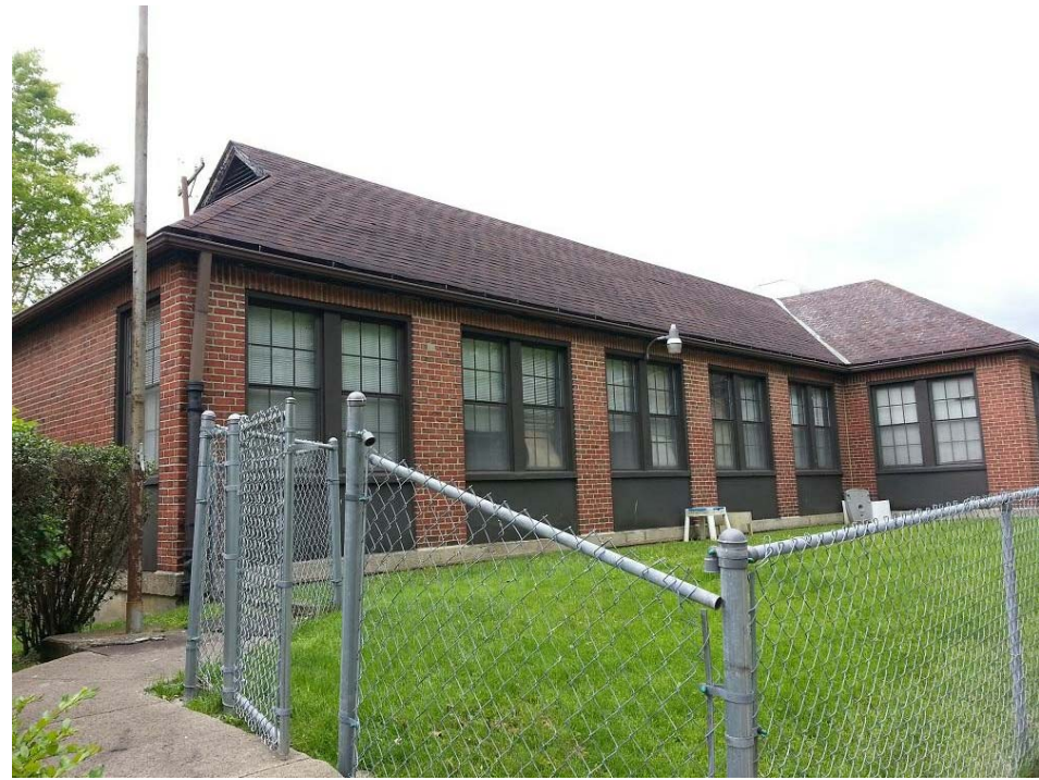
1 FRONT VIEWED FROM SOUTH - EAST
