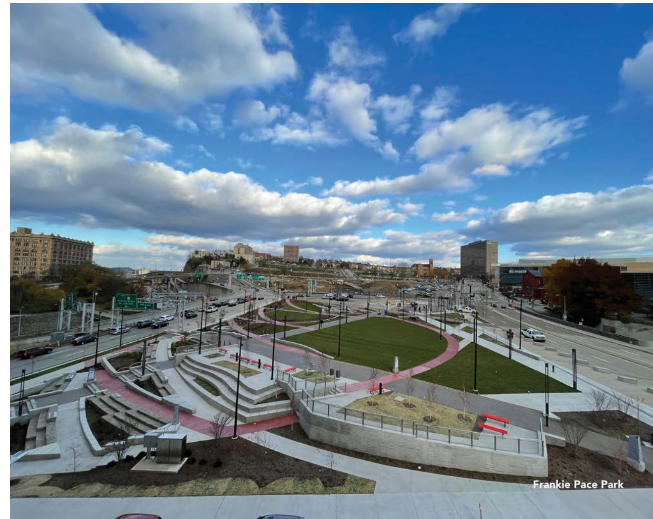
Figure 7.4 Aerial photo showing the constructed Frankie Mae Pace Park
