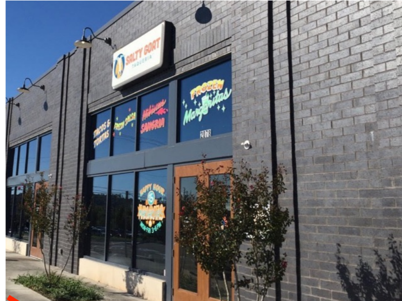
Brick Details on Facade
