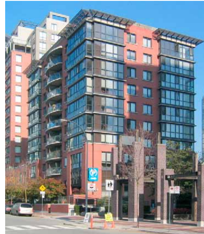
FIGURE 4.11 Example of how vertical bays are articulated through a change in materials, and a change in plane.
