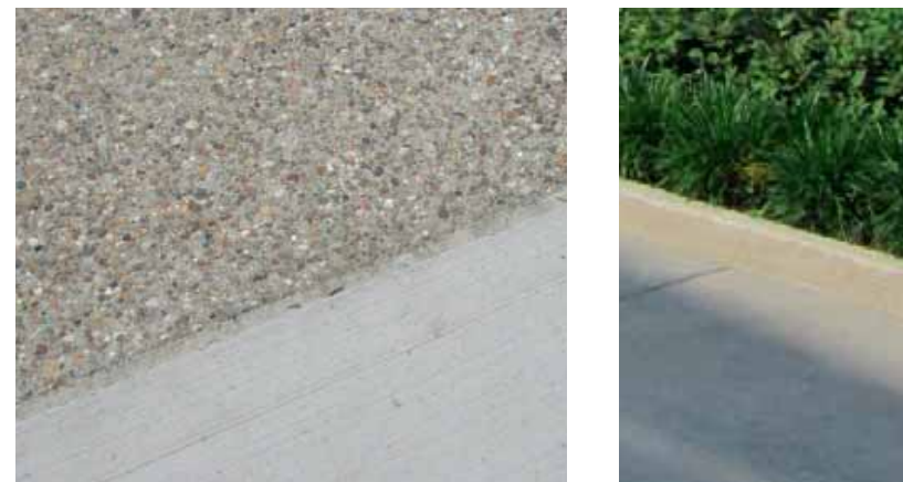
FIGURE 6.30 Example of exposed aggregate paving, broom finish concrete paving, and concrete planter curb.
