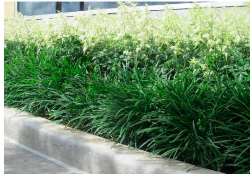
FIGURE 6.29 Example of concrete planter curb, planting bed, and broom finish concrete sidewalk
