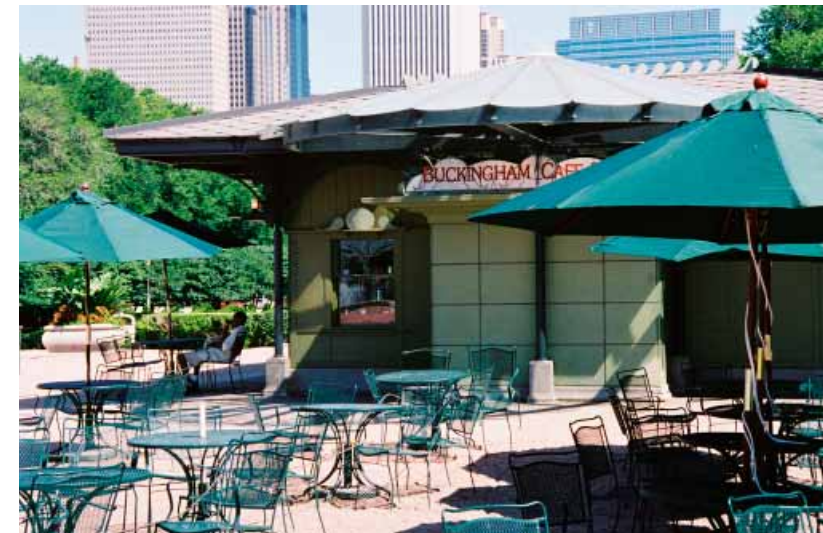
FIGURE 6.41 Example of moveable table/chairs and umbrellas appropriate for Parks and Open Space and Development Blocks
