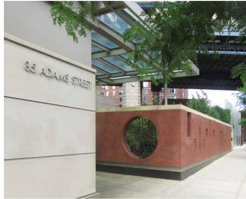
FIGURE 7.35 Typical commercial/residential frontage showing a recessed entry and walled garden beyond
