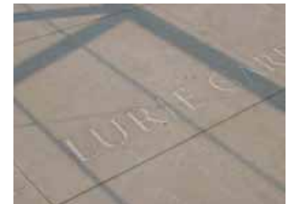
FIGURE 6.15 Example of paving enhanced with identity signage
