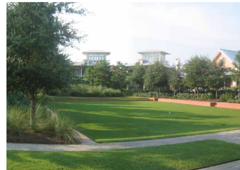
FIGURE 8.57 Passive stormwater retention occurs at this recessed lawn where rain can gradually infiltrate
