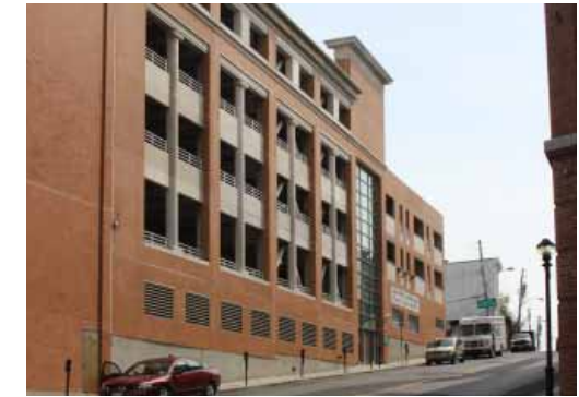
FIGURE 2.41 Example of a garage facade that is designed as if it were a building facade.
