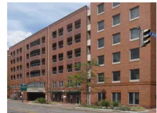
FIGURE 2.43 Example of a parking garage with conditioned spaces lining the end and ground floor.
