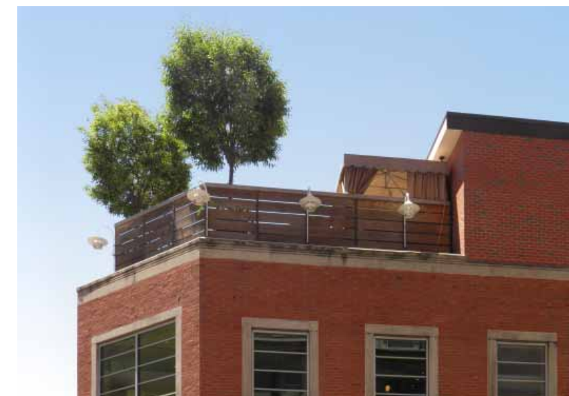
FIGURE 4.5 Example of a small penthouse that provides access to a rooftop terrace.
