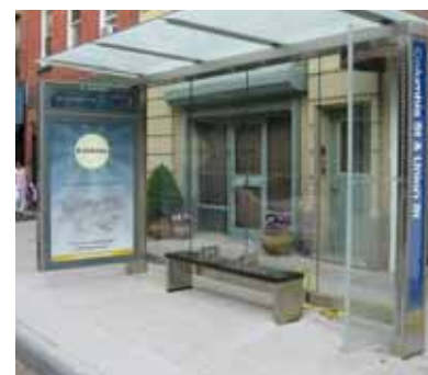
FIGURE 6.39 Example of bus shelter
