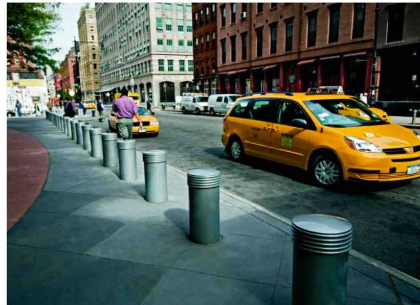
FIGURE 6.38 Example of security bollards (Landscape Forms)
