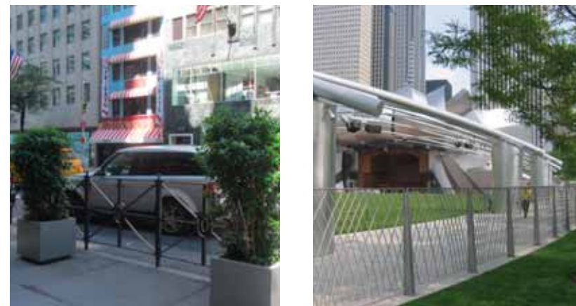
FIGURE 6.35 Example of barrier railings to control pedestrian traffic
