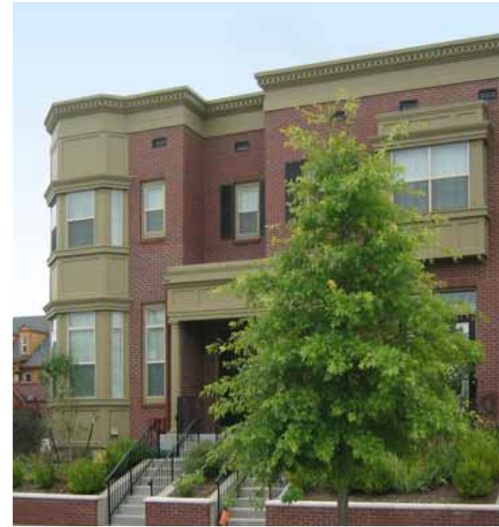
FIGURE 4.8 Attached Houses may have an elevated entry to provide some separation from street activity
