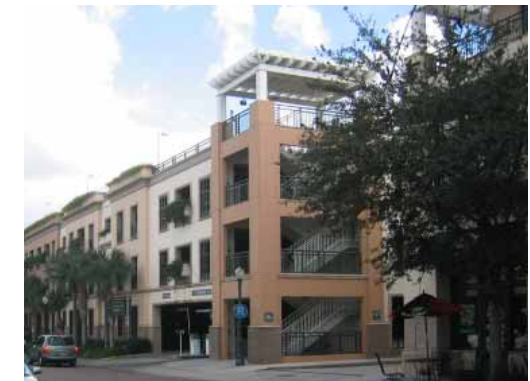
FIGURE 2.42 Examples of varying ways to treat parking garage facades along the street. Often corner elements may be emphasized as circulation locations.
