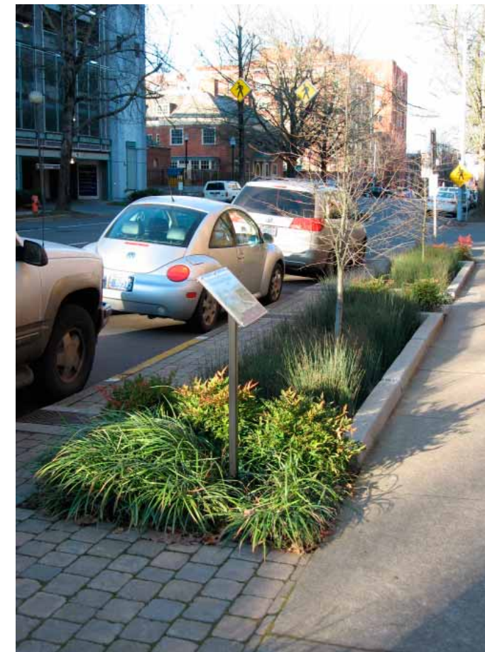
FIGURE 1.10 Example of a sustainable street design that contributes to reducing off-site runoff.
