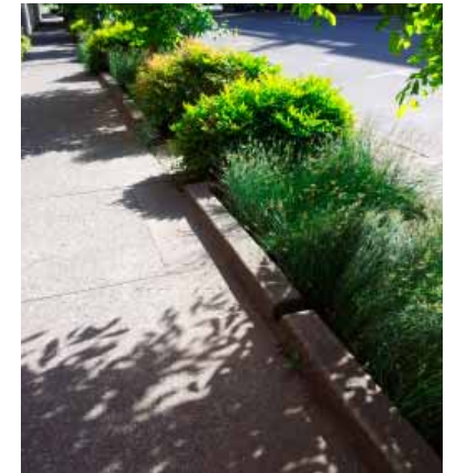
FIGURE 2.9 Curb cuts in planters allow stormwater runoff to enter infiltration planting pits.
