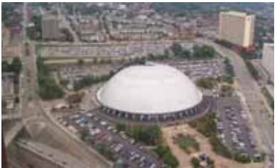
FIGURE 1.15 The Civic Arena pre-demolition
