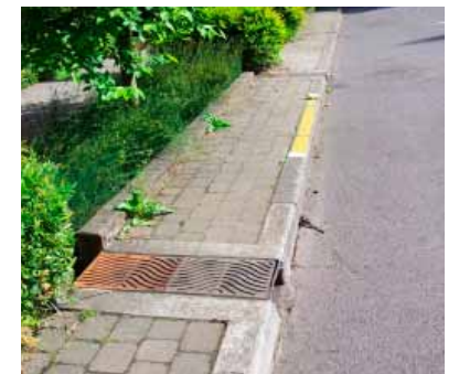
FIGURE 2.10 Decorative grates cover flush curbs allowing street runoff to enter infiltration planting pits.
