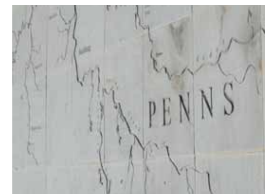
FIGURE 7.25 Example of environmental art. The water course is etched into the paving providing information of the surrounding region and pedestrian interest.
