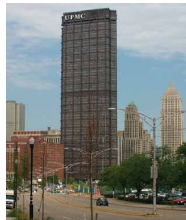
FIGURE 2.5 Context for Sub District 2
