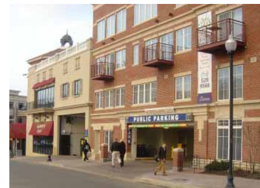
FIGURE 2.40 Example of podium parking where parking is entered off the street, and residential uses are stacked above the parking. Note how the architectural treatment of the building disguises the parking.
