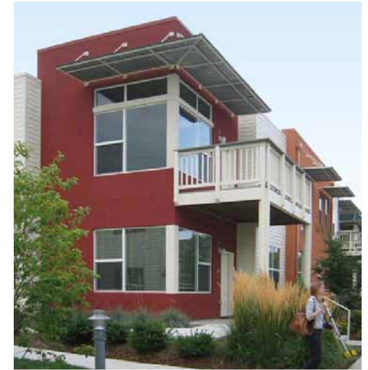
FIGURE 4.9 On end units corners may be emphasized through wrapping windows or wrap around porches
