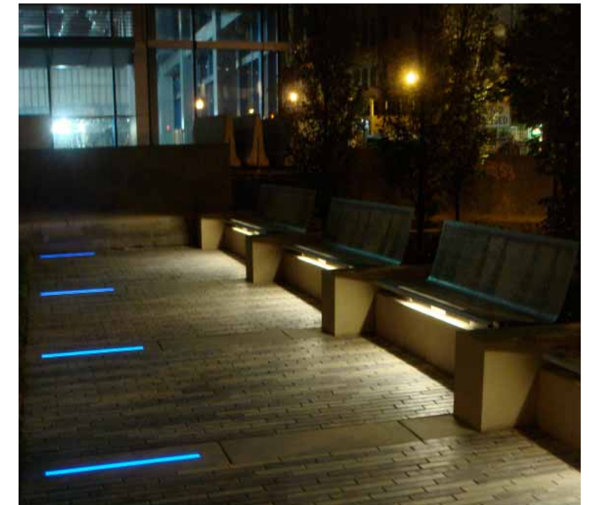
FIGURE 6.26 Example of LED pavement lighting — this type of application would be appropriate in Parks and Open Space and in the Development Blocks.
