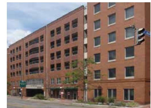
FIGURE 2.71 Example of a parking garage with conditioned spaces lining the end and ground floor.
