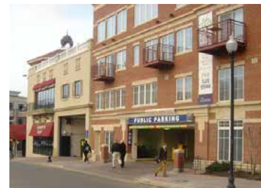
FIGURE 2.68 Example of podium parking where parking is entered off the street, and residential uses are stacked above the parking. Note how the architectural treatment of the building disguises the parking.
