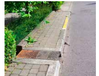
FIGURE 2.23 Decorative grates cover flush curbs allowing street runoff to enter infiltration planting pits.
