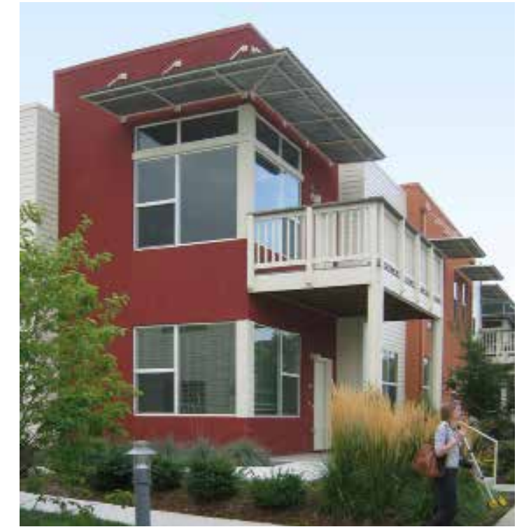
FIGURE 4.14 On end units corners may be emphasized through wrapping windows or wrap around porches.
