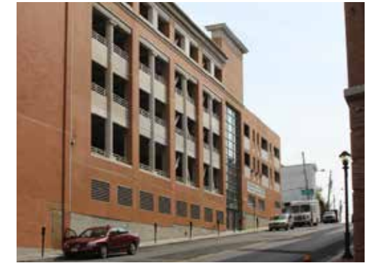
FIGURE 2.69 Example of a garage facade that is designed as if it were a building facade.
