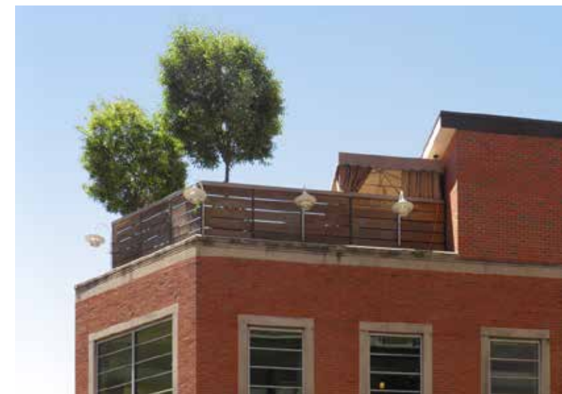
FIGURE 4.10 Example of a small penthouse that provides access to a rooftop terrace.
