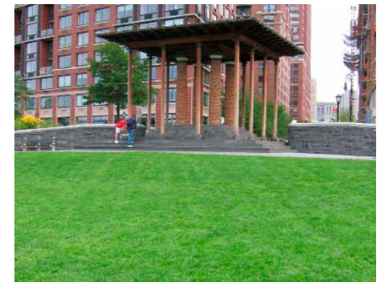
FIGURE 7.21 Pavilions along lawn areas provide relief from the sun.
