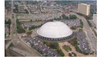
FIGURE 1.11 The Civic Arena pre-demolition
