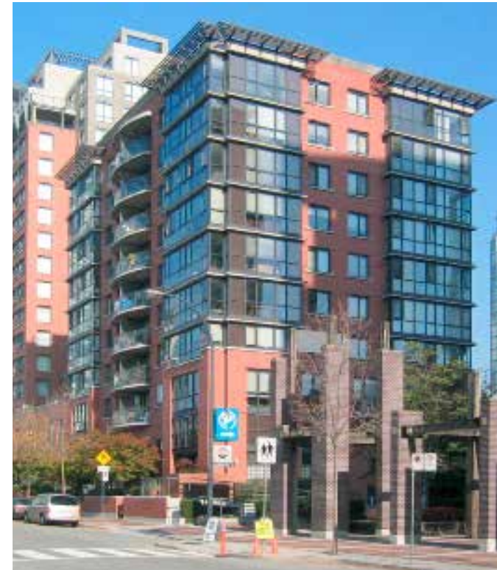
FIGURE 4.18 Example of how vertical bays are articulated through a change in materials, and a change in plane.
