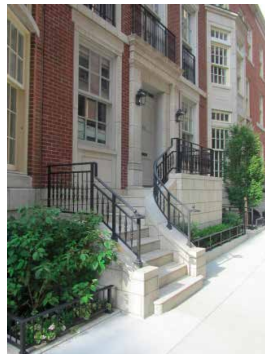
FIGURE 2.47 Typical residential frontage showing planting beds with fencing at edge of walks
