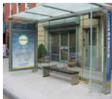
FIGURE 6.18 Example of bus shelter.
