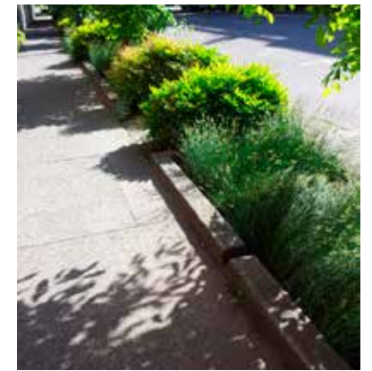
FIGURE 2.22 Curb cuts in planters allow stormwater runoff to enter infiltration planting pits.
