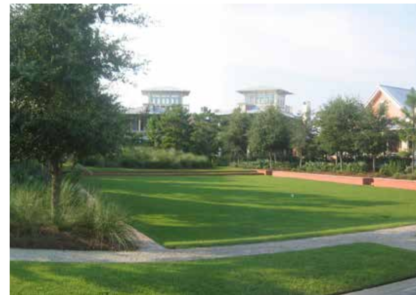
FIGURE 2.13 Passive stormwater retention occurs at this recessed lawn where rain can gradually infiltrate
