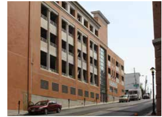
FIGURE 2.69 Example of a garage facade that is designed as if it were a building facade.
