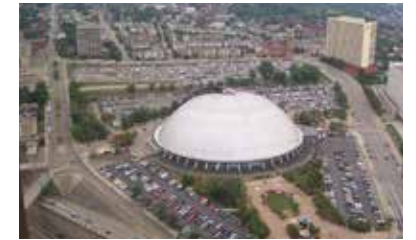
FIGURE 1.11 The Civic Arena pre-demolition
