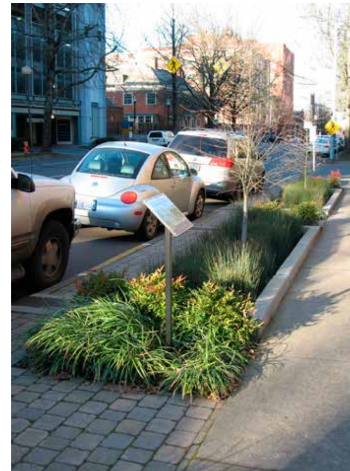
FIGURE 1.8 Example of a sustainable street design that contributes to reducing off-site runoff.
