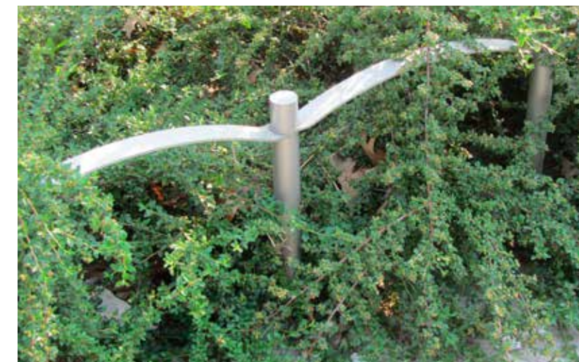
FIGURE 3.41 Example of tree planter protection fence in addition to planter curb for high traffic areas.
