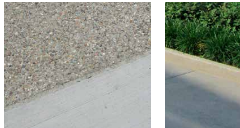
FIGURE 3.39 Example of exposed aggregate paving, broom finish concrete paving, and concrete planter curb.
