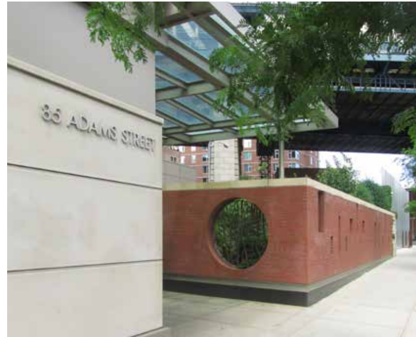
FIGURE 2.44 Typical commercial/residential frontage showing a recessed entry and walled garden beyond
