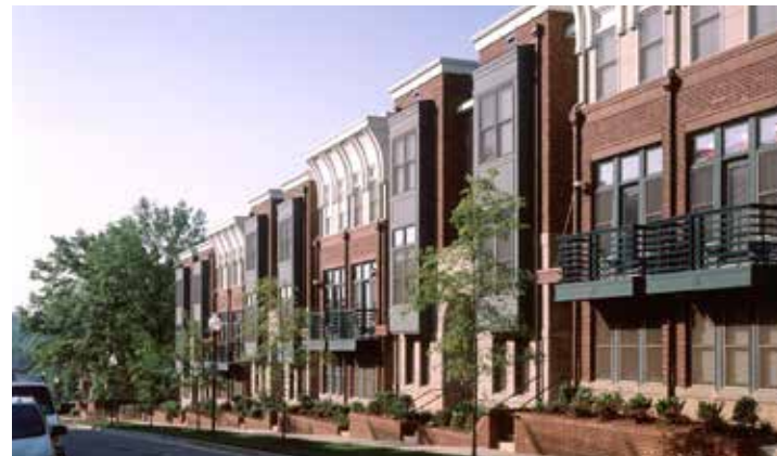
FIGURE 4.15 Example of Type I building in a townhouse form with decorative bays and balconies
