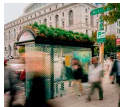
FIGURE 6.19 Example of bus shelter with a Green Roof.
