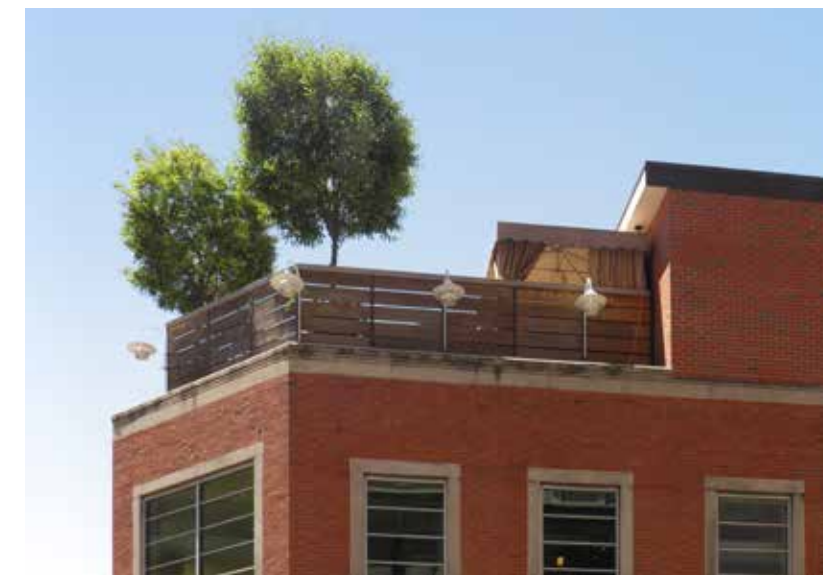
FIGURE 4.10 Example of a small penthouse that provides access to a rooftop terrace.
