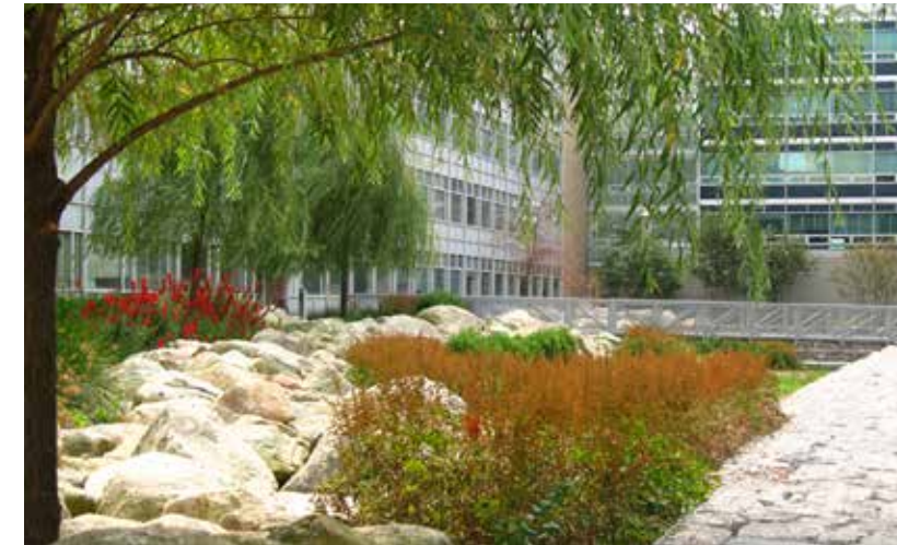
FIGURE 2.8 Stormwater retention area with native plantings and gabion walls
