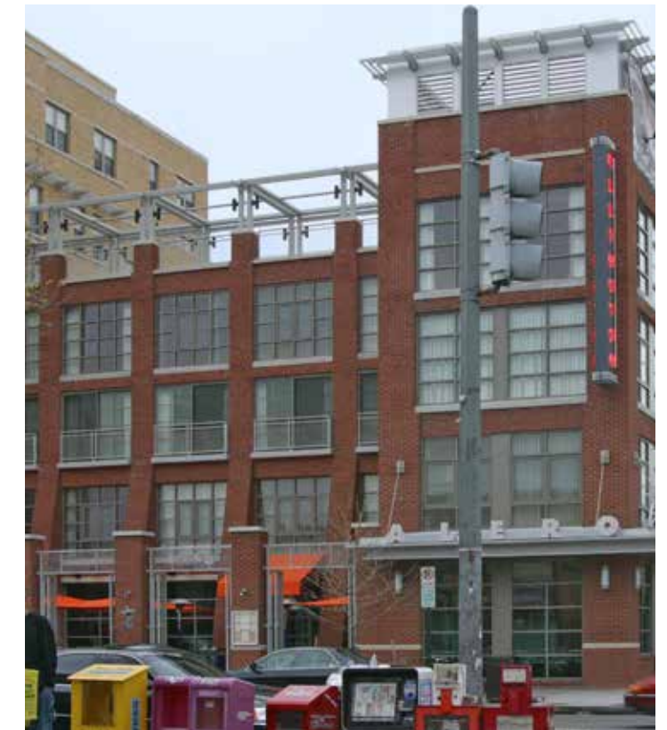
FIGURE 4.19 Corner elements enhance the composition of a building and may also be used to terminate vistas.
