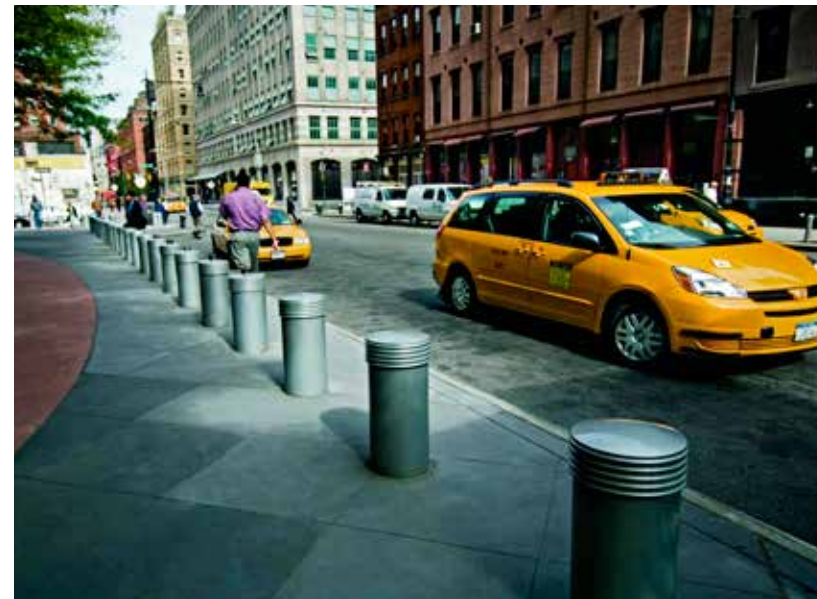
FIGURE 6.17 Example of security bollards (Landscape Forms).
