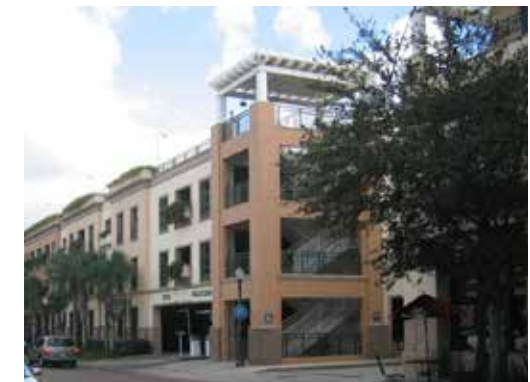
FIGURE 2.70 Examples of varying ways to treat parking garage facades along the street. Often corner elements may be emphasized as circulation locations.
