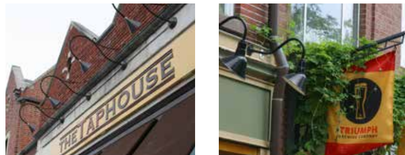
FIGURE 6.7 Examples of wall mounted lighting
