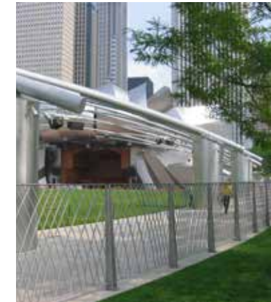
FIGURE 6.16 Example of contemporary, art-influenced barrier railings.
