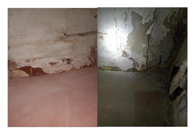
6.3 West Foundation Wall: it was observed during the inspection that the West foundation wall had been replaced with concrete blocks at some point. This should be noted since the replacement of the sandstone foundation with a new concrete block wall resulted from a deficiency that had to be mitigated. And if the root cause has not been addressed, this type of deficiency will continue in the foundation structure. Reference the picture below taken during the inspection.
