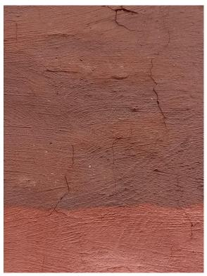
6.7 West Building Exterior: On the building's West side, at some point, a stucco covering was applied to it more recently than the east side. This wall appears to be in better shape than the exterior walls. However, there are signs of moisture running down the face as a result of poor downspouts or coping above, plus there are signs of moisture getting underneath the stucco, as shown where it has fallen off the side of the building. Reference the pictures below for these deficiencies.
