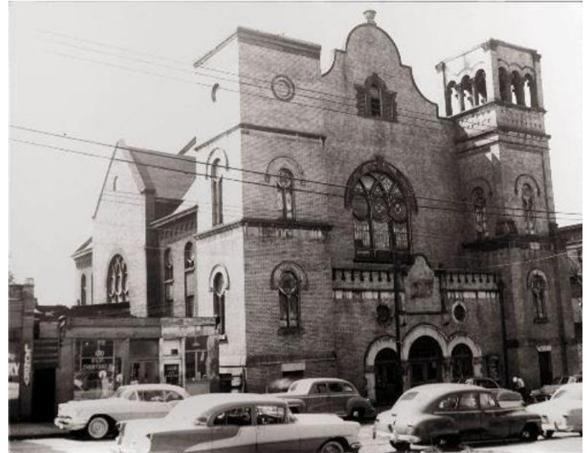
Historic Bethel Prior to Demolition
