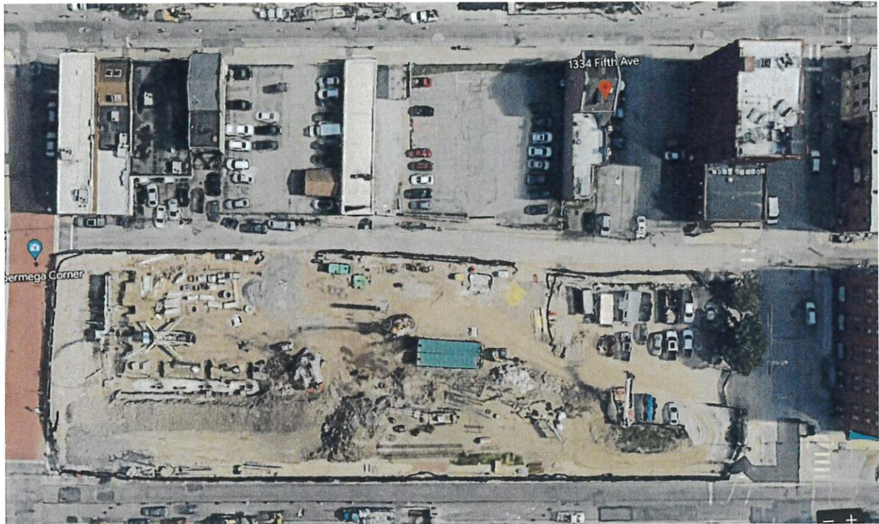
Google Earth image with location marked at Subject Property. Fifth Avenue is at the top of the image. Orbital Engineering is the rightmost building, located on the corner of Fifth and Stevenson. Orbital Employee parking is located to the left of the Orbital Engineering building. Subject Property is marked and is to the left of the Orbital employee parking lot.
