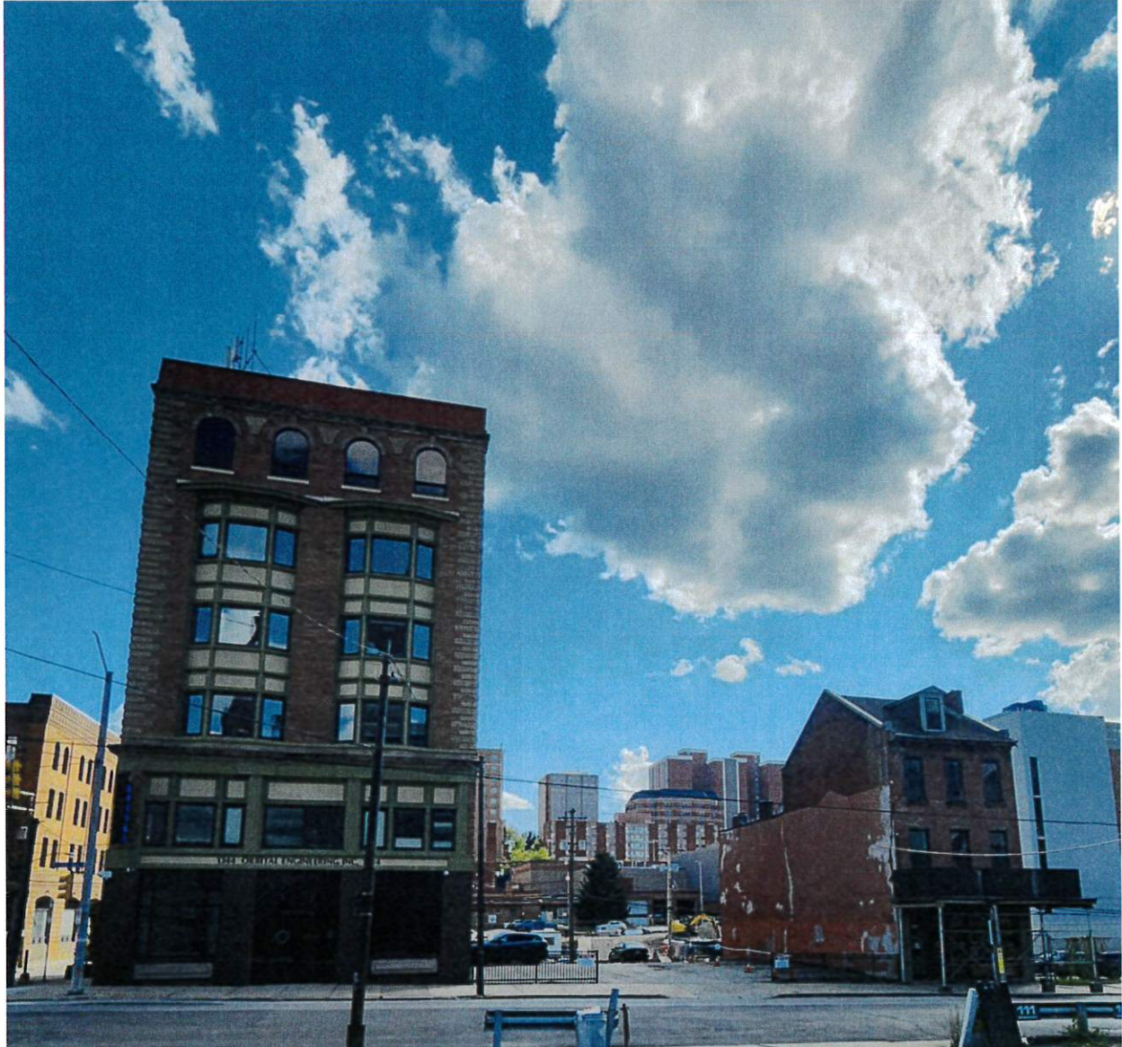
Orbital Engineering (1344 Fifth Ave) pictured left, employee parking in center, Subject Property (1334 Fifth Ave) pictured right.
